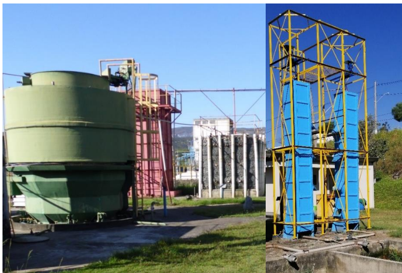
FIGURE III.1.2 – UASB reactor (green to the left size) and biological filters (blue in the right)
